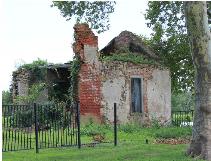
The remnants of the original Herrman's family house constructed at around 1660, located at the Bohemia Manor Farm vineyards near the Bohemia River
